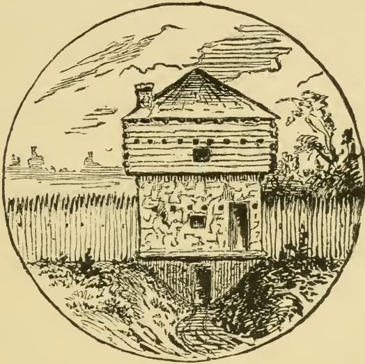
Block House, Built in 1780.
